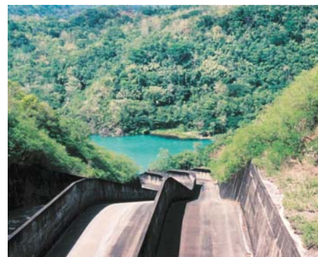
Angat spillway, another key to maintaining public water supply in the Philippines.
