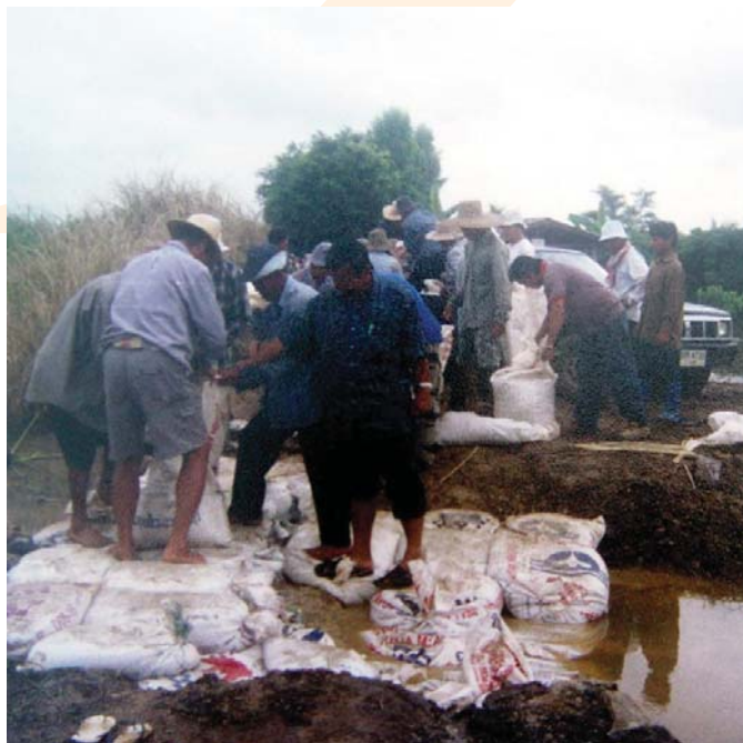
A collective action in MKT led by the headman to build the community sandbag dike.
