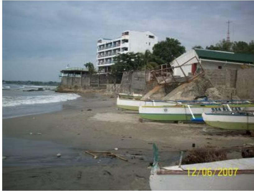
Figure 8. Bulkheads in San Fernando Bay
