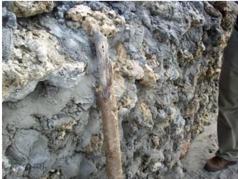
Figure 9. Bulkhead constructed from rocks and sand sourced from the beach
