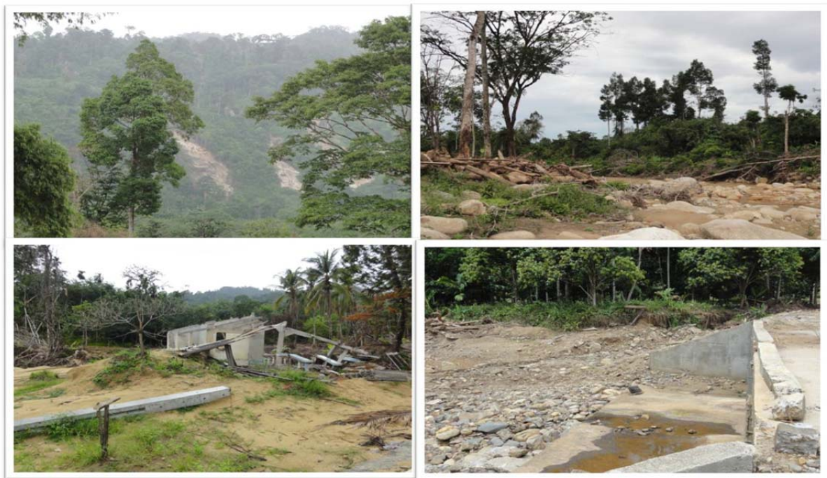
Figure 1. Damages from flash flood during March-April 2011 (Nakhon Si Thammarat)
