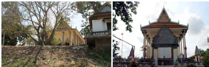
Figure 13. Preak Kmeng temple (left) in Preak Kmeng commune, and Peam Ta Erk temple (right) in Preak Oknha Ong commune,
