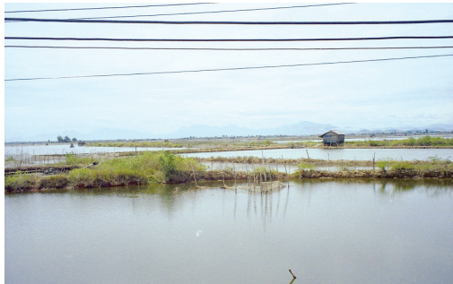
Dikes contribute to wetland degradation in Vietnam's Mekong River Delta.
